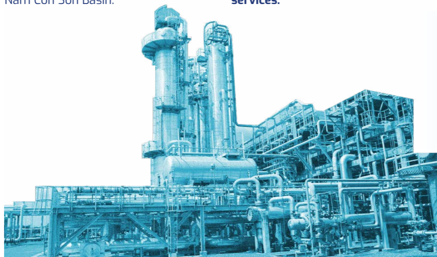
Dinh Co Gas Processing Plant Project (08/2001 - 02/2002)
