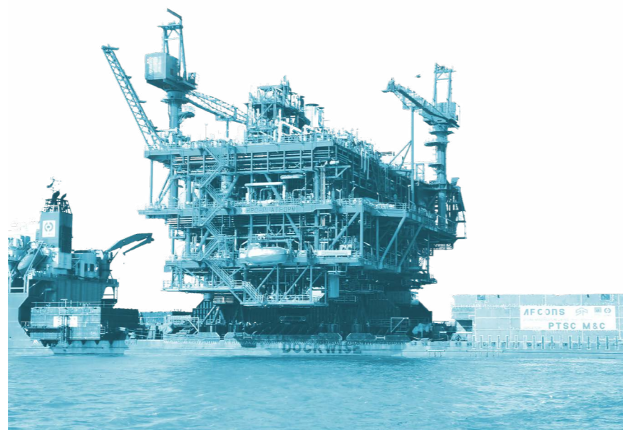
The HRD Offshore Platform Topside
